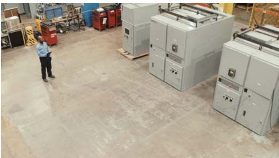
Remote circuit breaker racking. Credit: Eaton.
