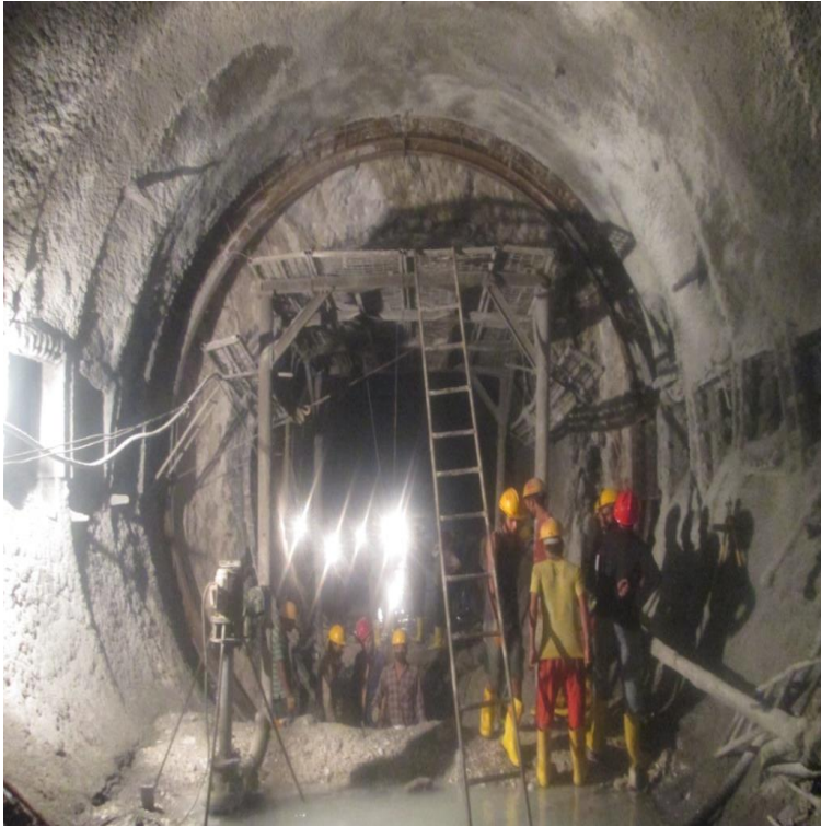
NEW STEEL RIB INSTALLATION
