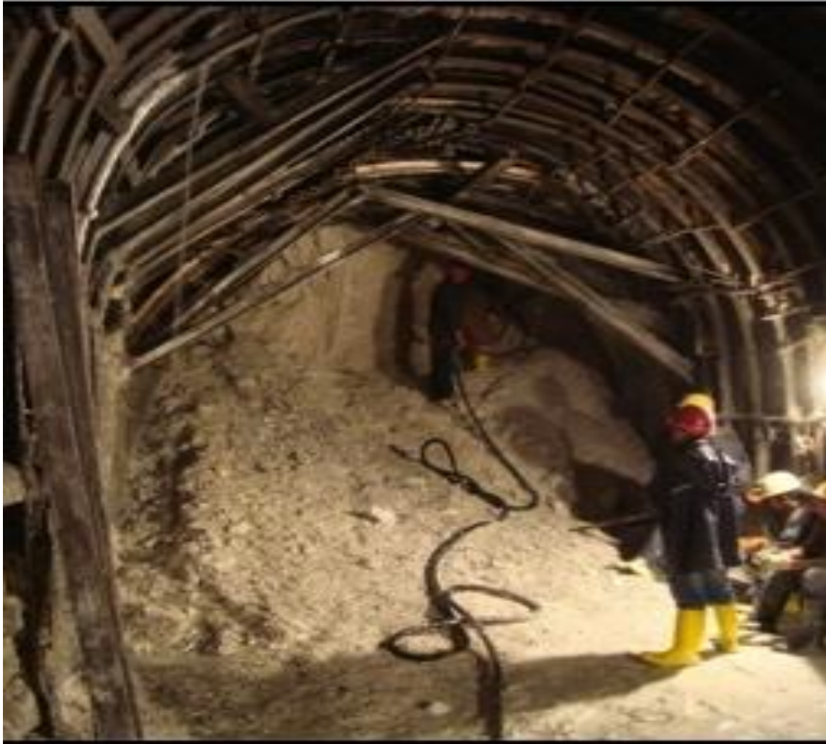
TUNNEL SQUEEZING
