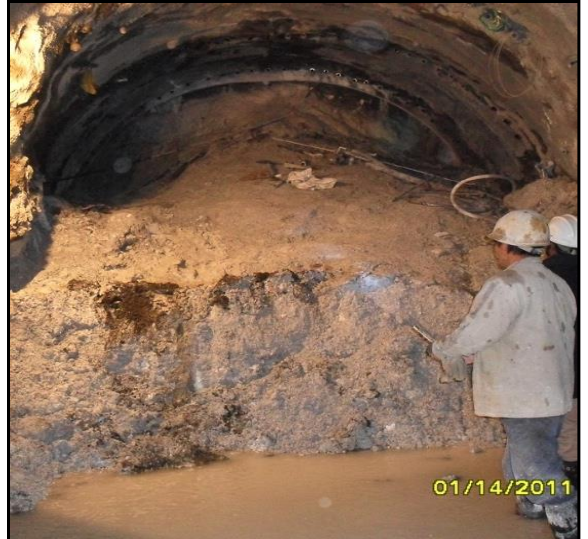
MUD FLOW AFTER SQUEEZING
