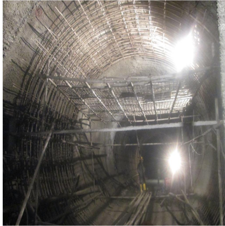
NEW STEEL BAR INSTALLATION
