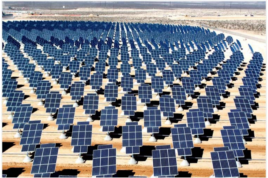
Nellis Solar Power Plant, in Nellis Air Force Base, northeast of Las Vegas.
